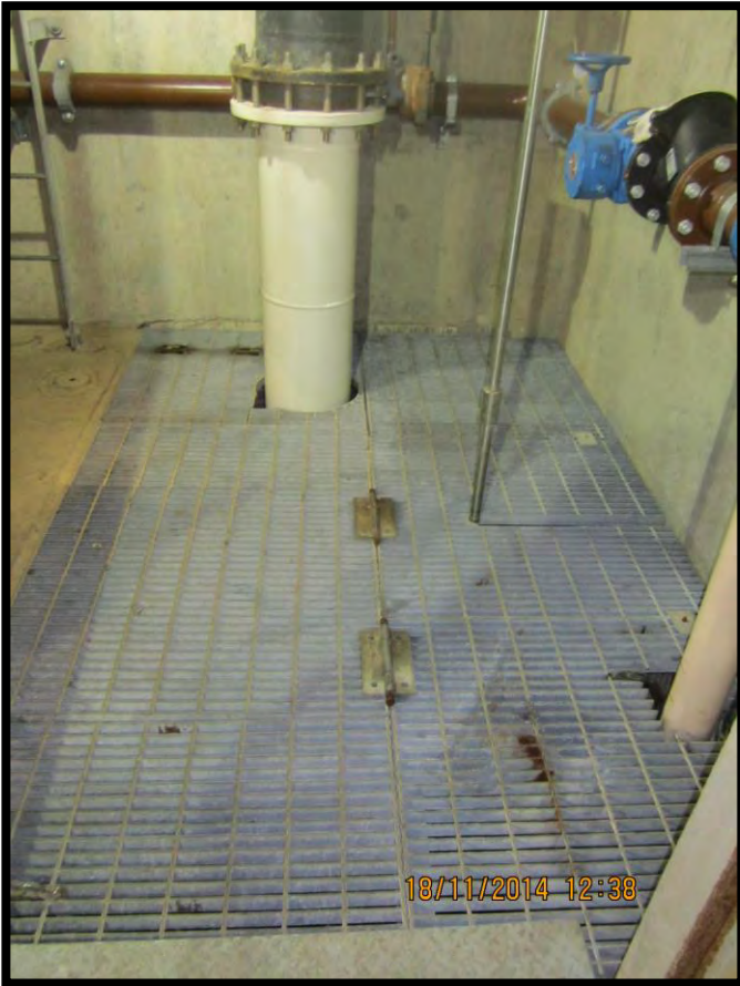
Intake Well Access Landing
