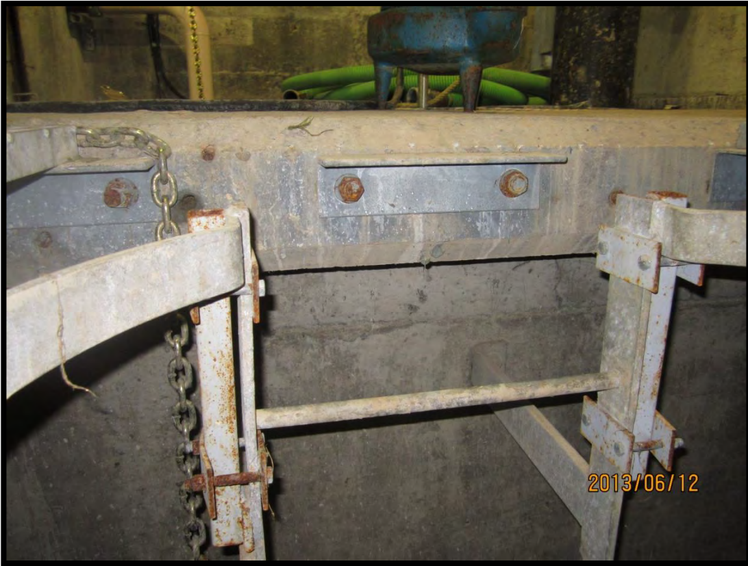
Typical Ladder Rung
