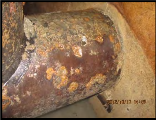
Raw Water Intake Lines Prior to 2014 Replacement
