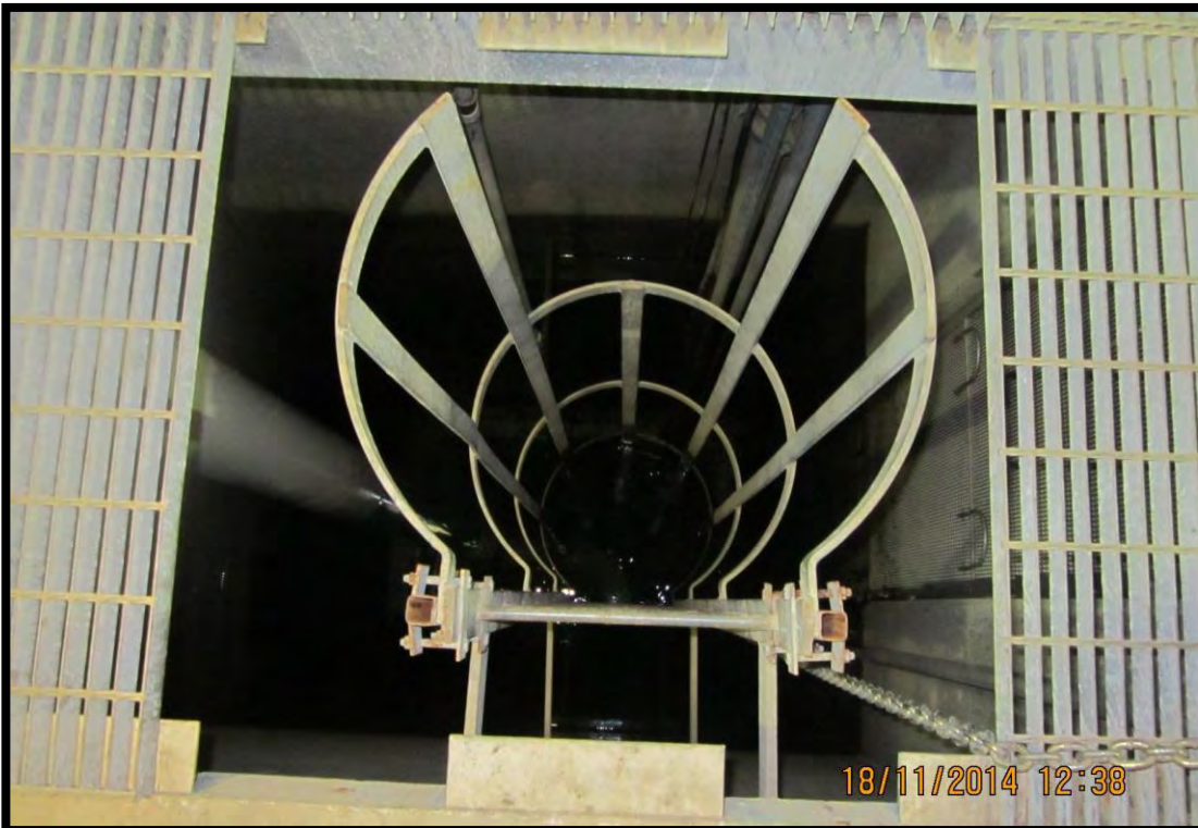
Intake well access ladder entry
