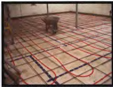
Preparation of Floor
