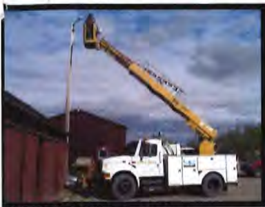
Yard Light Installation
