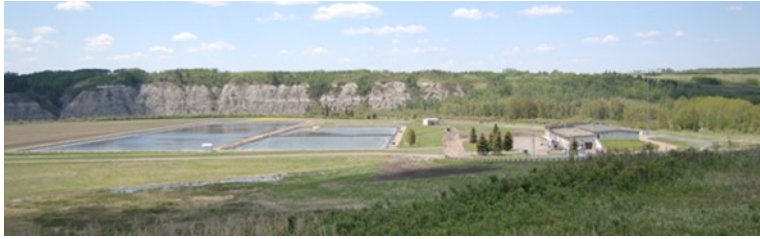
Raw water reservoirs
