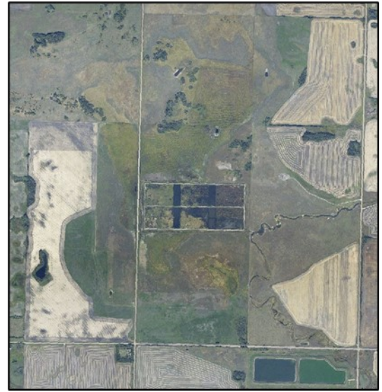
Arial view of waste water treatment
