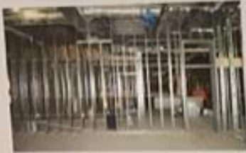
Standard Building pre/post drywall
