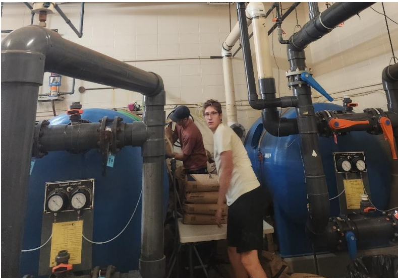
Carter helping out the Contractor with the sand bags
