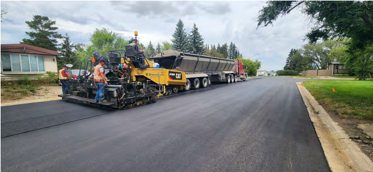
Spruce Grove paving (shown above)
