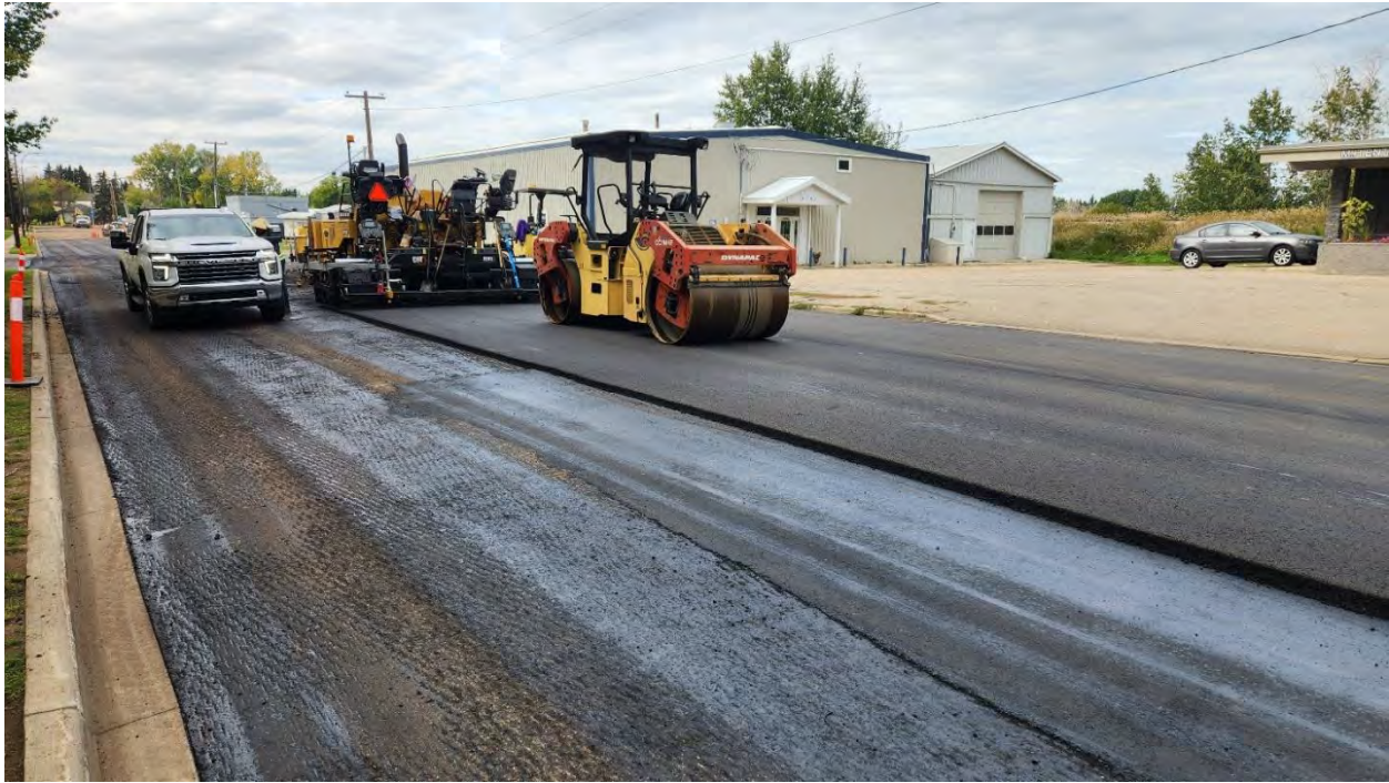
Highway 56 paving (shown above)
