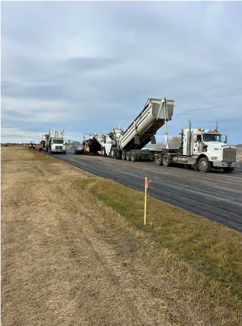
Airport Paving (shown above)
