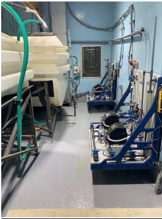
Finished Containment Area 3
