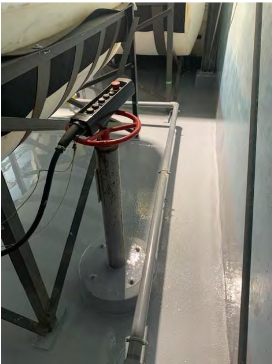
Finished Containment Area 2
